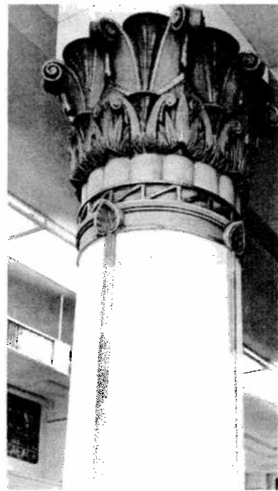
One of the column capitals in the Reebie Storage Warehouse.
